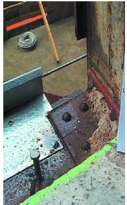
Above and below: At 550 West Jackson, a project in Chicago, problems were encountered when an existing slab was being modified. Existing columns interfered with embed locations.
