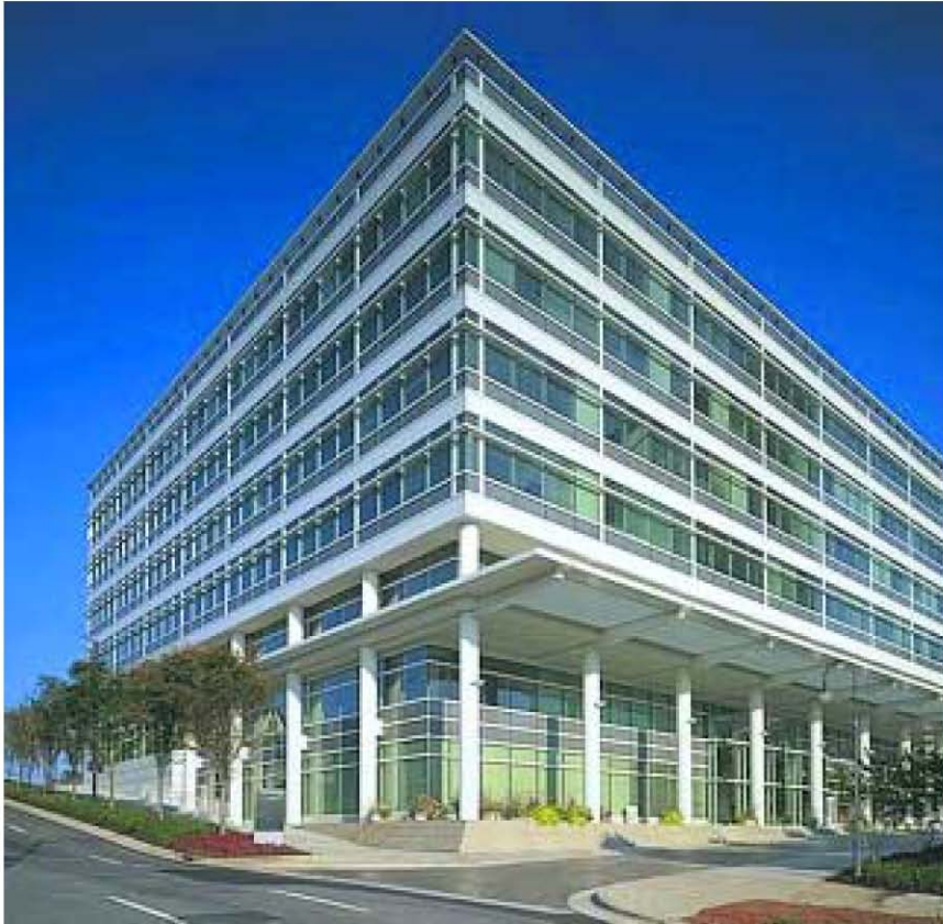
The Wachovia Building in North Carolina is an example of a successfully detailed curtain wall system.
