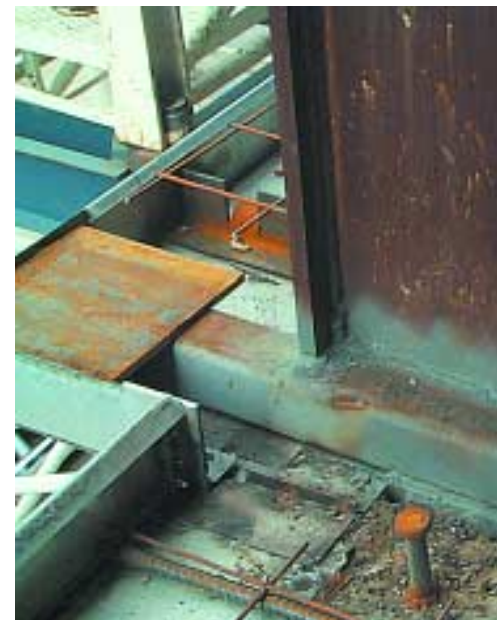
Above and below: At 550 West Jackson, a project in Chicago, problems were encountered when an existing slab was being modified. Existing columns interfered with embed locations.
