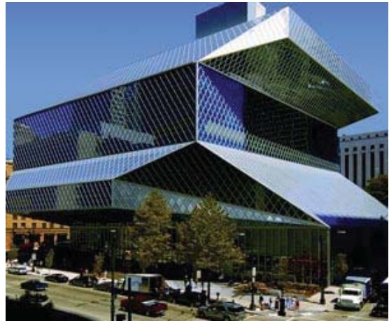
Proper attention to and utilization of the appropriate technical standards has contributed to the lasting performance of the Seattle Central Library's façade.
